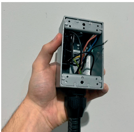
2 Note the location of the wires. Disconnect and remove the wires from the junction box. Refer to Fig. 2 for junction box wiring diagram.
