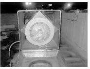
7.) Drain the accumulated waste water from the fan. If necessary, remove one of the drain plugs from the grease trap. Dispose of waste water correctly. Be sure to reinstall the drain plug when finished.
