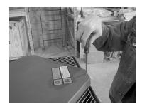
3.) Place the (4) 6 mm nuts onto the (4) motor mounting bolts.
